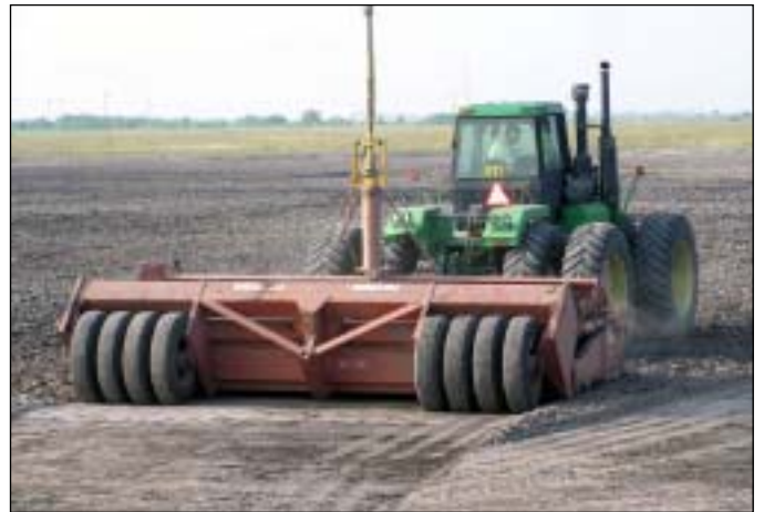
Figure 4. Pond construction using a laser-guided pan behind a tractor.
